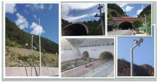
The EIC-CDP22E Photometer is a self contained intelligent analyser and the measurements are converted into an output signal of 4-20 mA (directly proportional to the luminance measurement).
